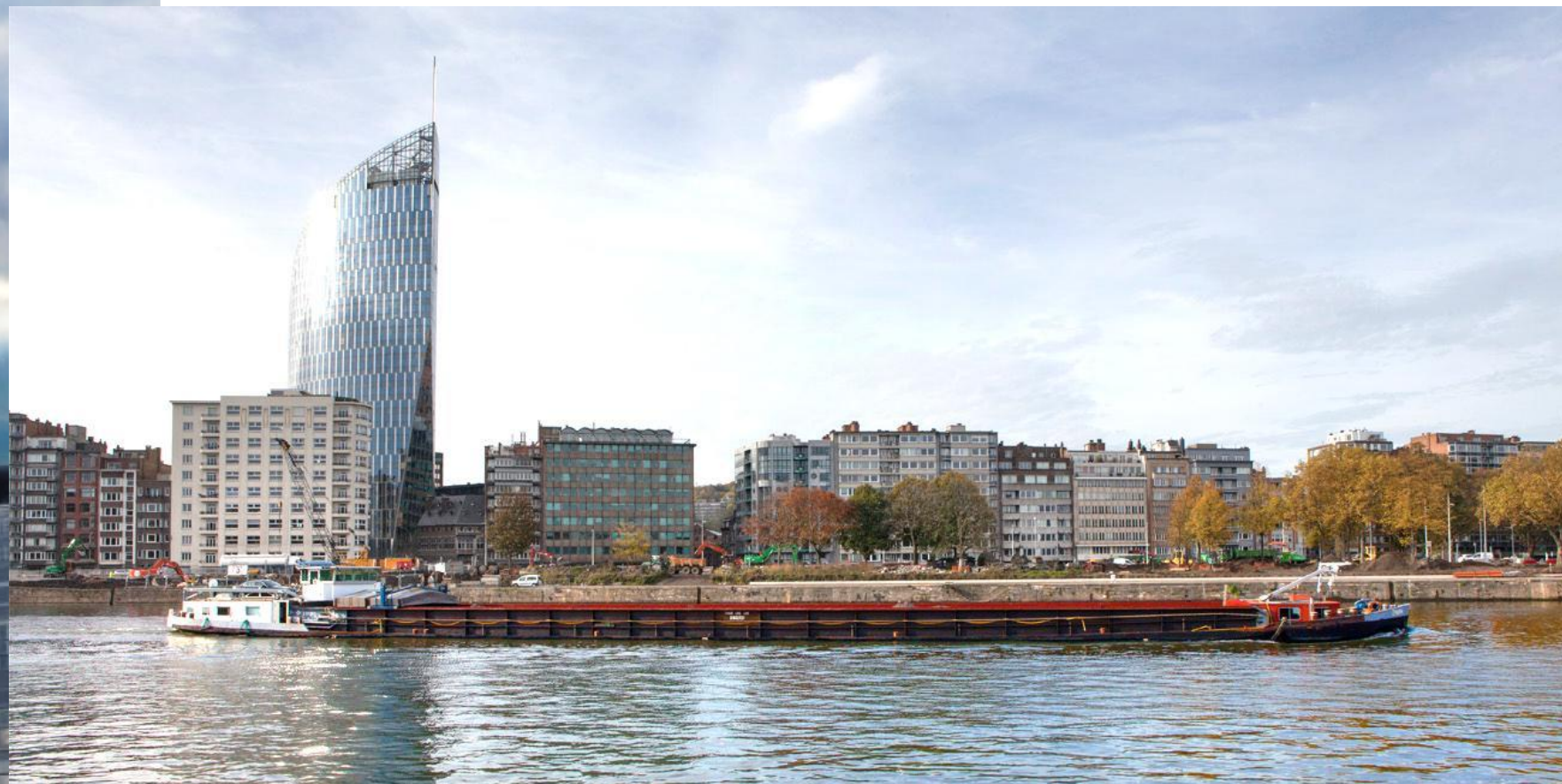
Tour des Finances Liège – Jaspers Eyers Architects – 126kWc
